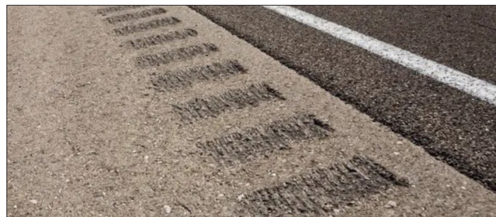
Figure 3. Short milled rumble strips adaptable to airport use. (Photo courtesy of the U.S. Department of Transportation Federal Highway Administration)
